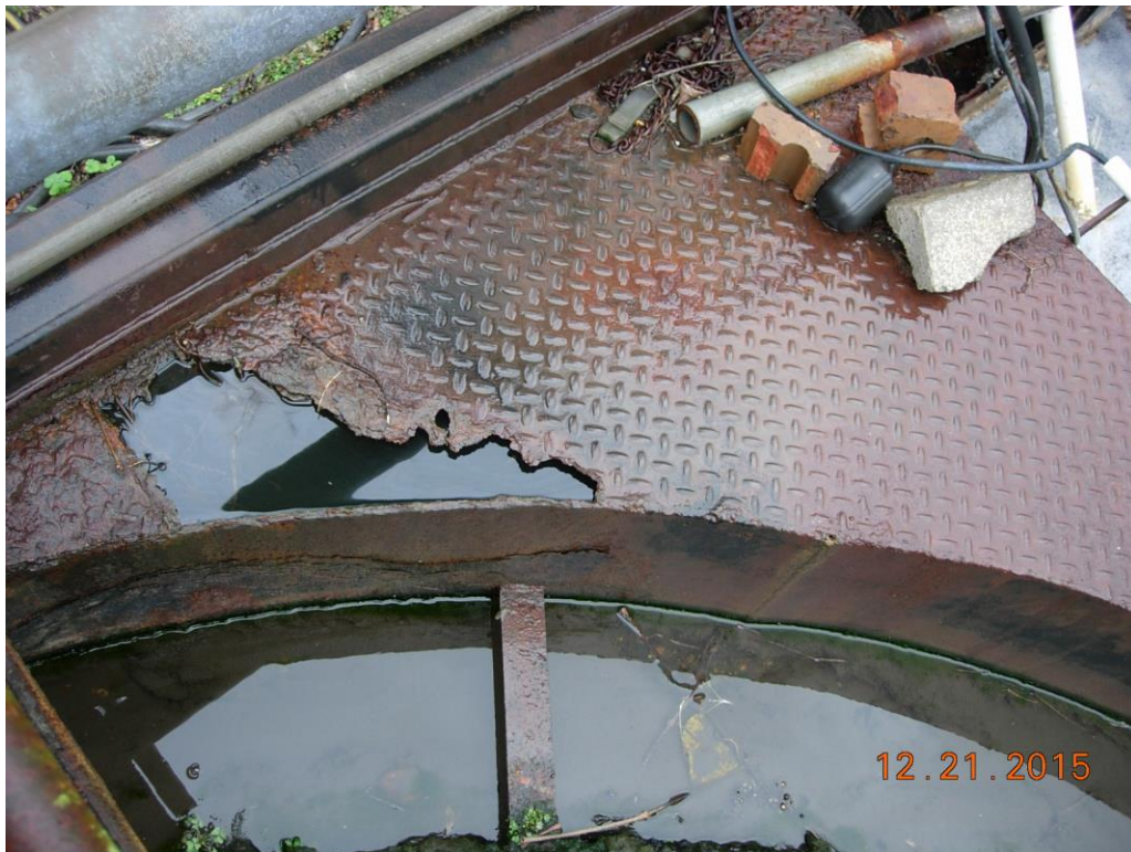
Severely corroded clarifier structure with hole in decking & with metal flaking off of weir trough
