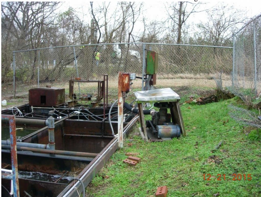
Single blower motor beside plant with flexible hose connection to air lines
