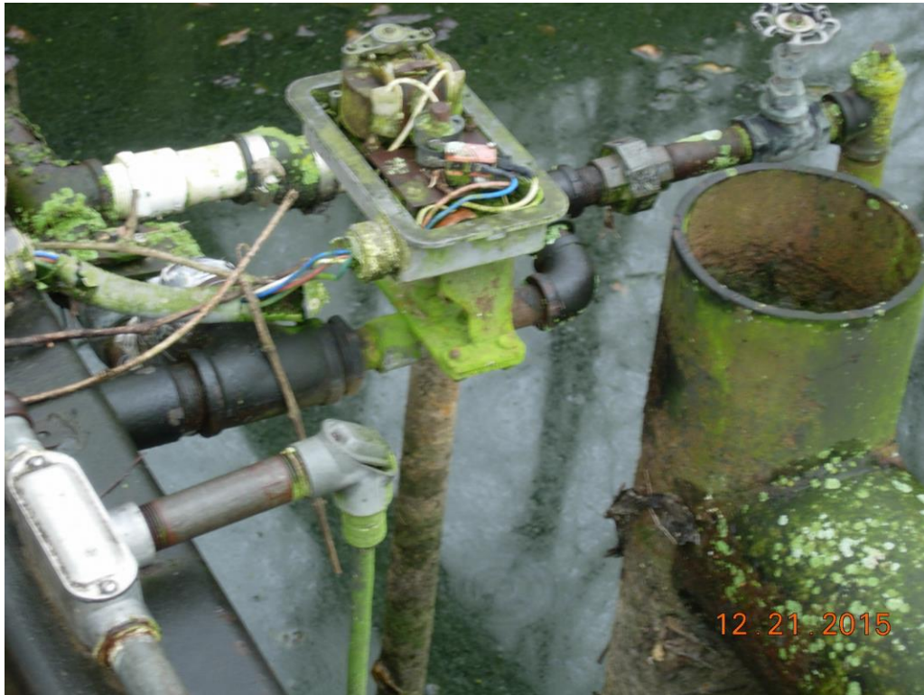
Deteriorated wiring conditions
