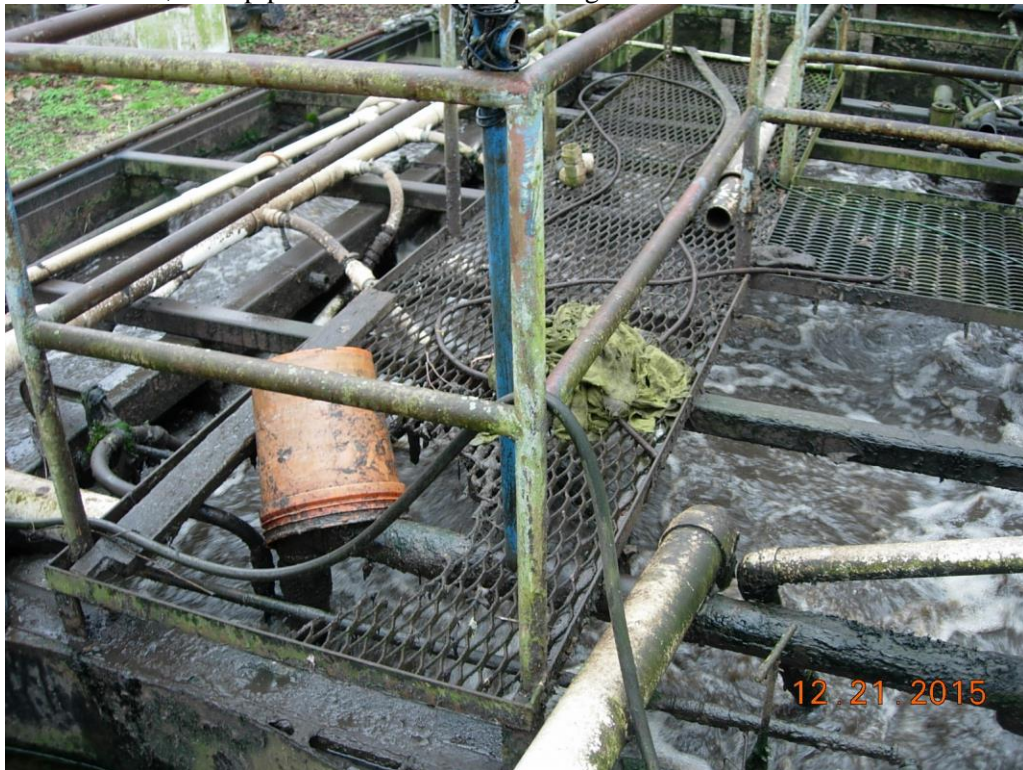
Aeration basin walkway corroded through around return sludge line, return sludge line covered with plastic bucket, rock & 2 x 4 on bucket & wedged under hand rails is used to hold bucket in place
