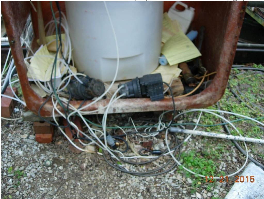
Chlorination solution & de-chlorination solution feed pumps, wiring, & feed lines
