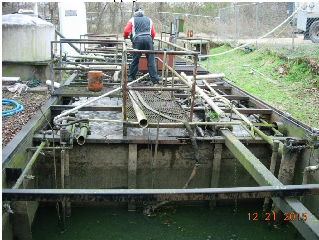
Digester & aeration basin, deteriorated/corroded metal structures & makeshift repairs of piping
