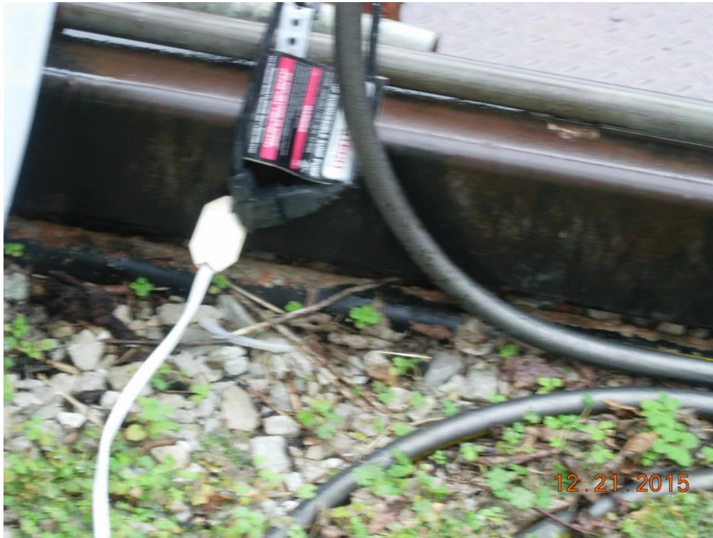
Example of extension cords used for wiring, exposed to wet weather & wastewater from treatment units
