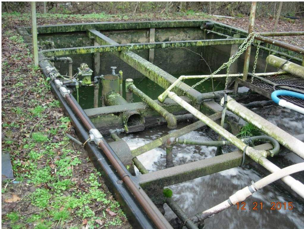
Deteriorated condition of structures, piping & wiring, makeshift repairs & replacement of metal piping with PVC and flexible hoses
