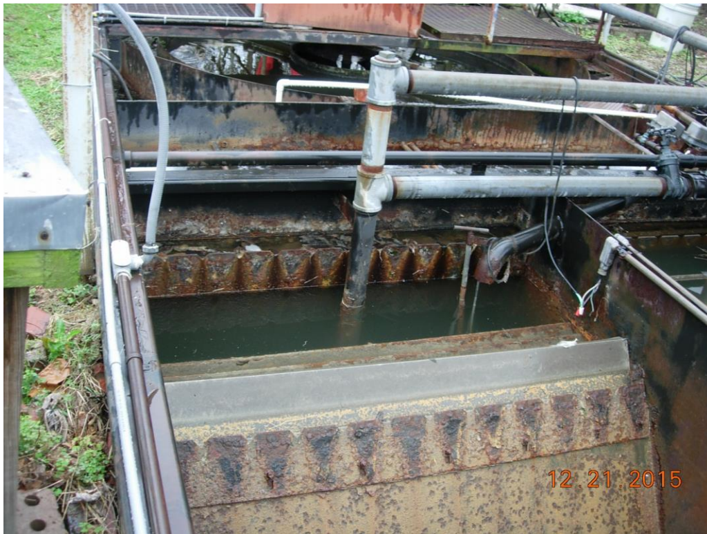
Corroded second filter structure & weir trough
