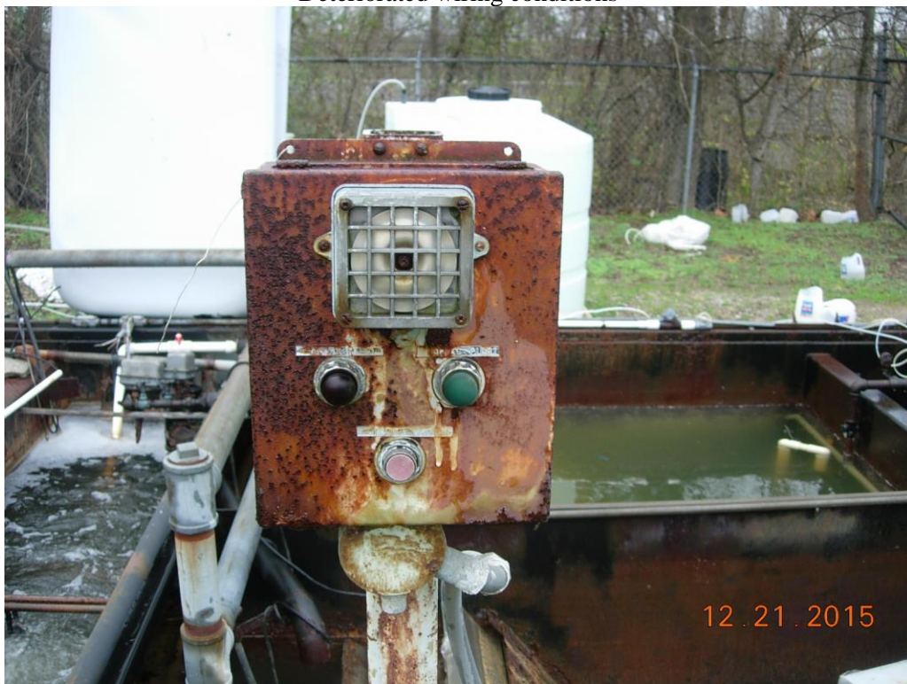
Deteriorated electrical system conditions
