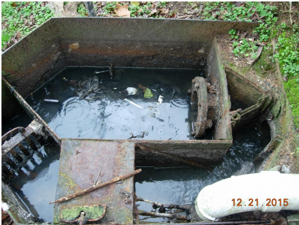
Influent bar screens showing severe corrosion, bar screens breaking apart & ineffective screening of raw wastewater
