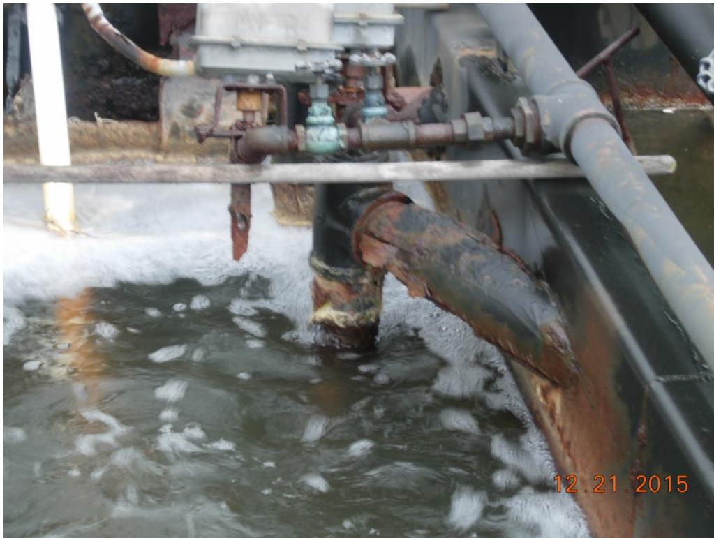
Corroded, broken piping, broom handle support
