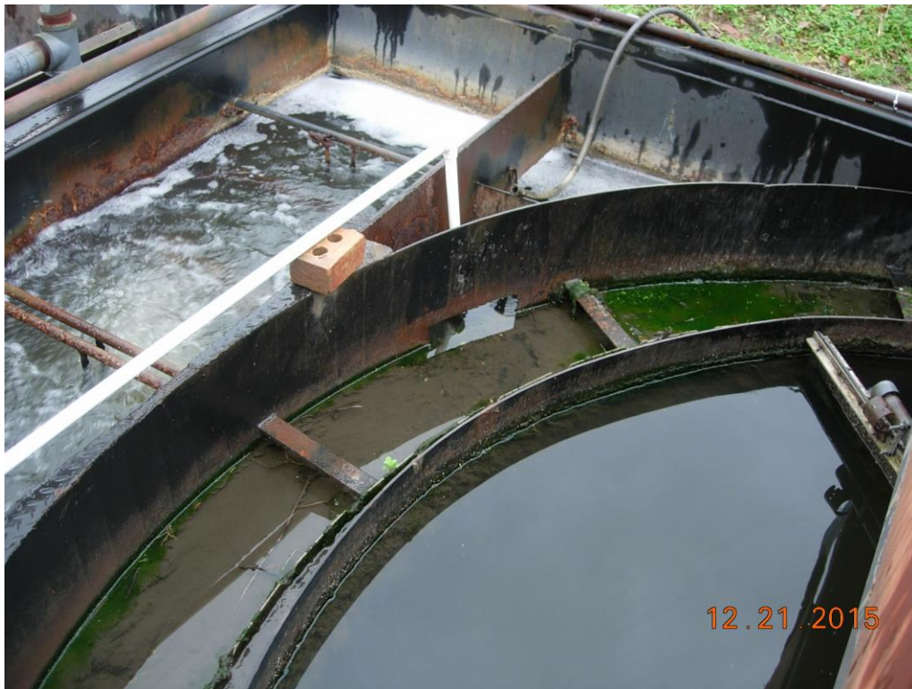
Clarifier with solids exiting weir trough
