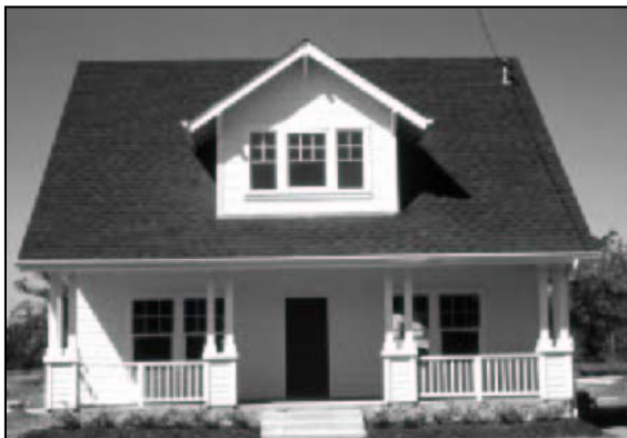
Figure 3-8 3-10: This house demonstrates vertically oriented windows, a raised foundation, and a front porch consistent with existing historic homes in CAO 2.
