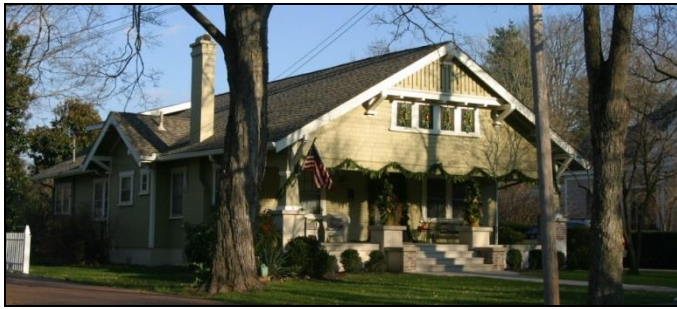
Figure 3-7 3-9: Example of a gabled roof with overhanging eaves as required in CAO 2.
