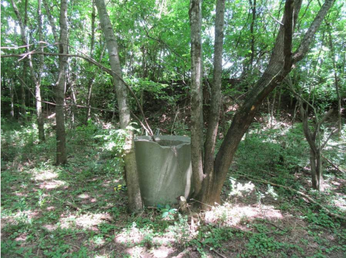
Photo No. 13: 36-inch-diameter RCP pipe downstream of dam.
