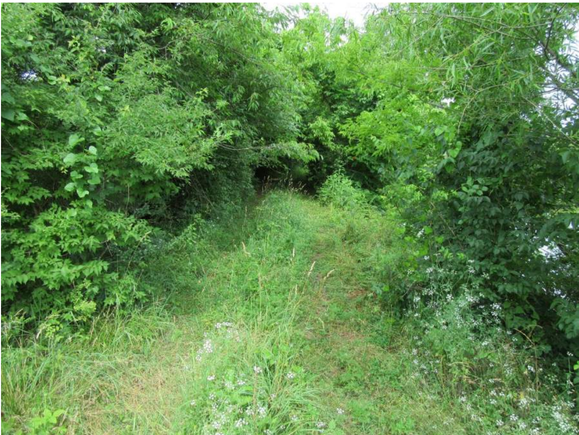
Photo No. 2: Crest viewed from left abutment.
