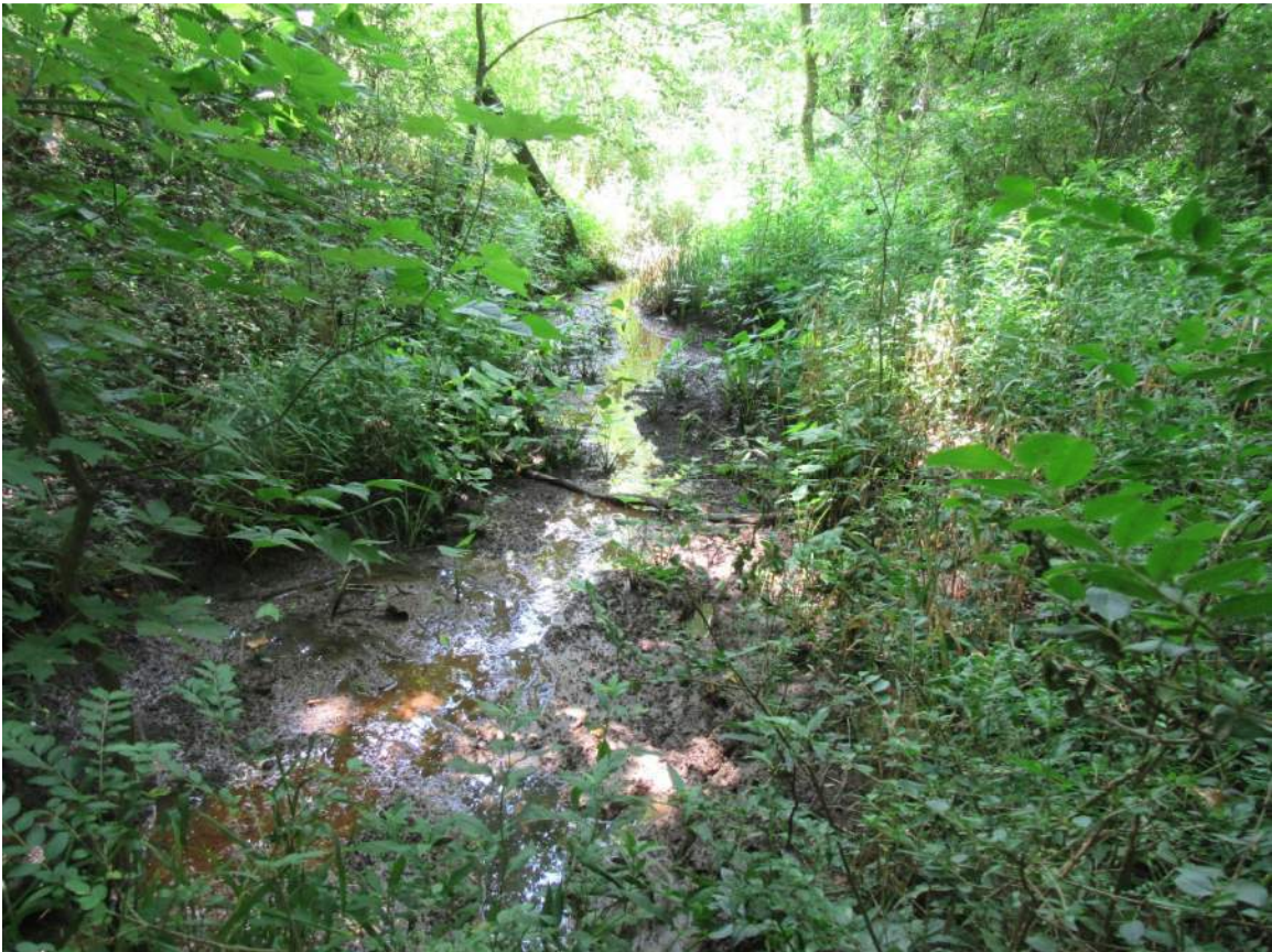
Photo No. 14: Seepage downstream of RCP pipe.
