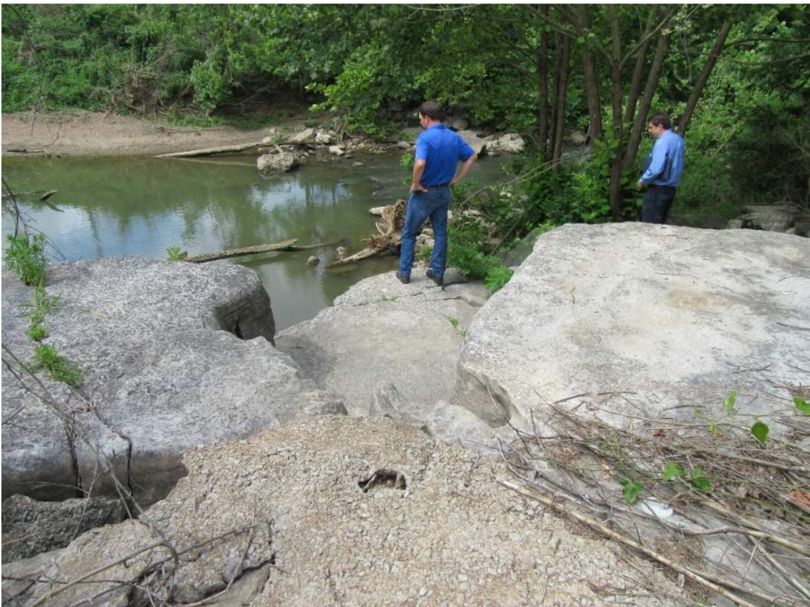
Photo No. 20: Bedrock drop-off at downstream end of spillway discharge channel.
