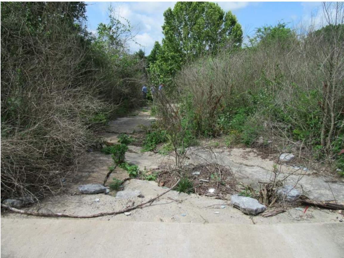
Photo No. 18: Spillway discharge channel viewed looking downstream.
