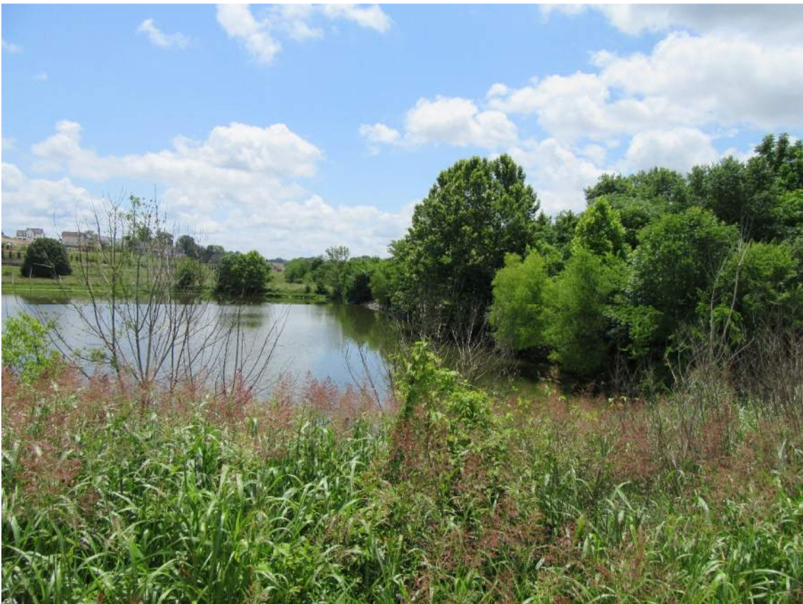
Photo No. 6: Upstream slope viewed from right abutment.
