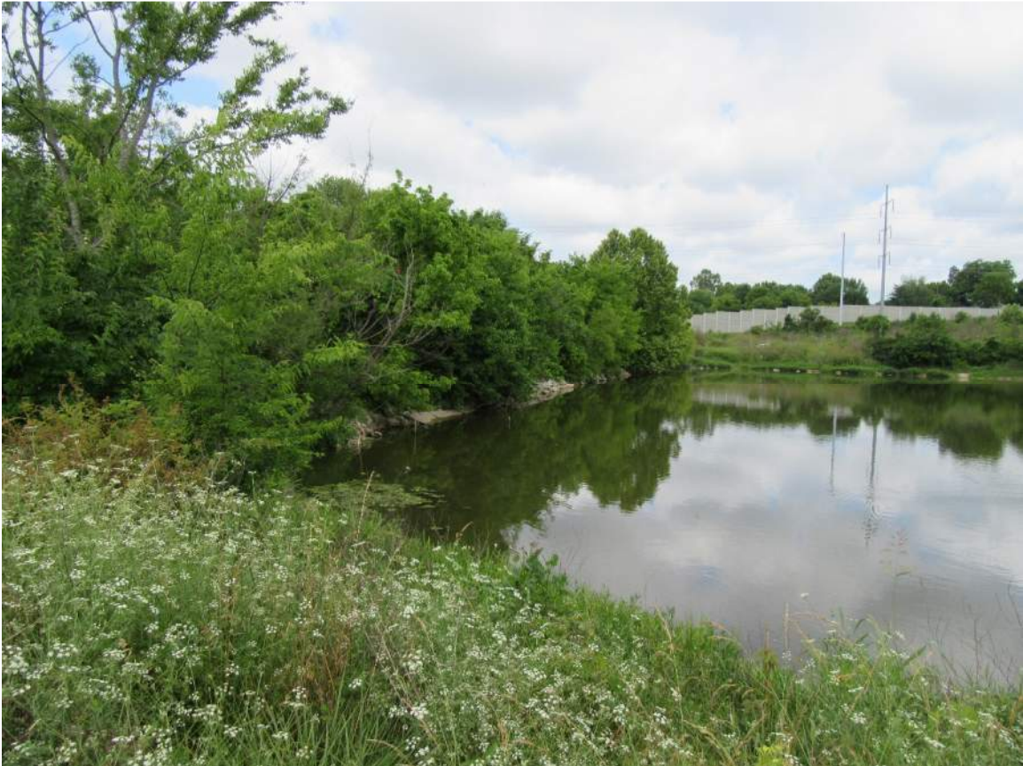
Photo No. 5: Upstream slope viewed from left abutment.
