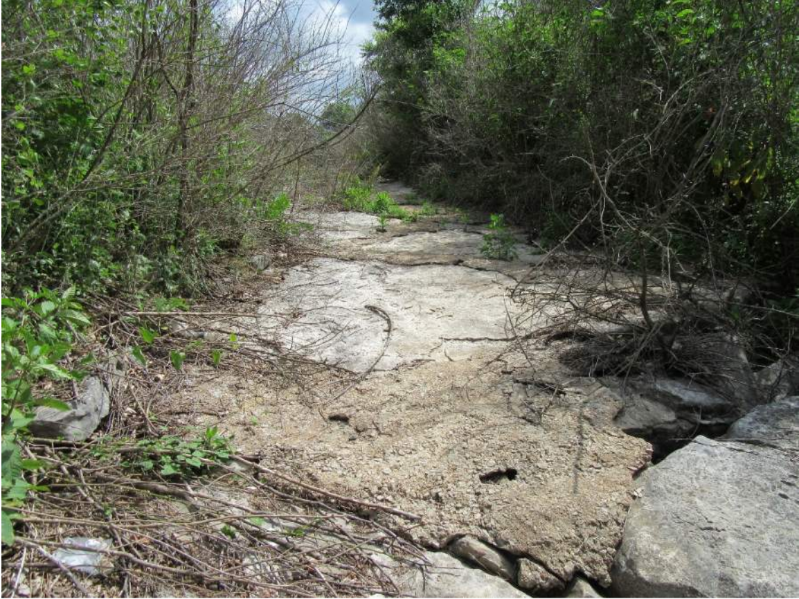
Photo No. 19: Spillway discharge channel viewed looking upstream.
