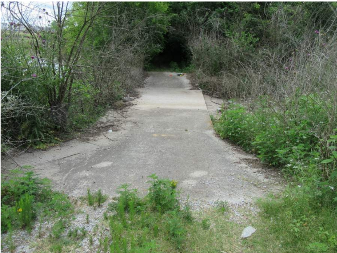
Photo No. 16: Spillway weir viewed from right abutment.
