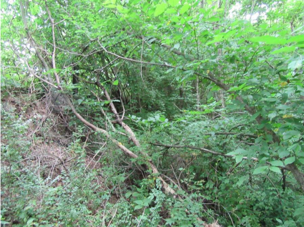
Photo No. 9: Downstream slope viewed from right abutment.
