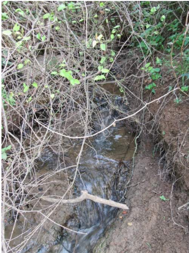
Photo No. 22: Seepage to left of spillway.
