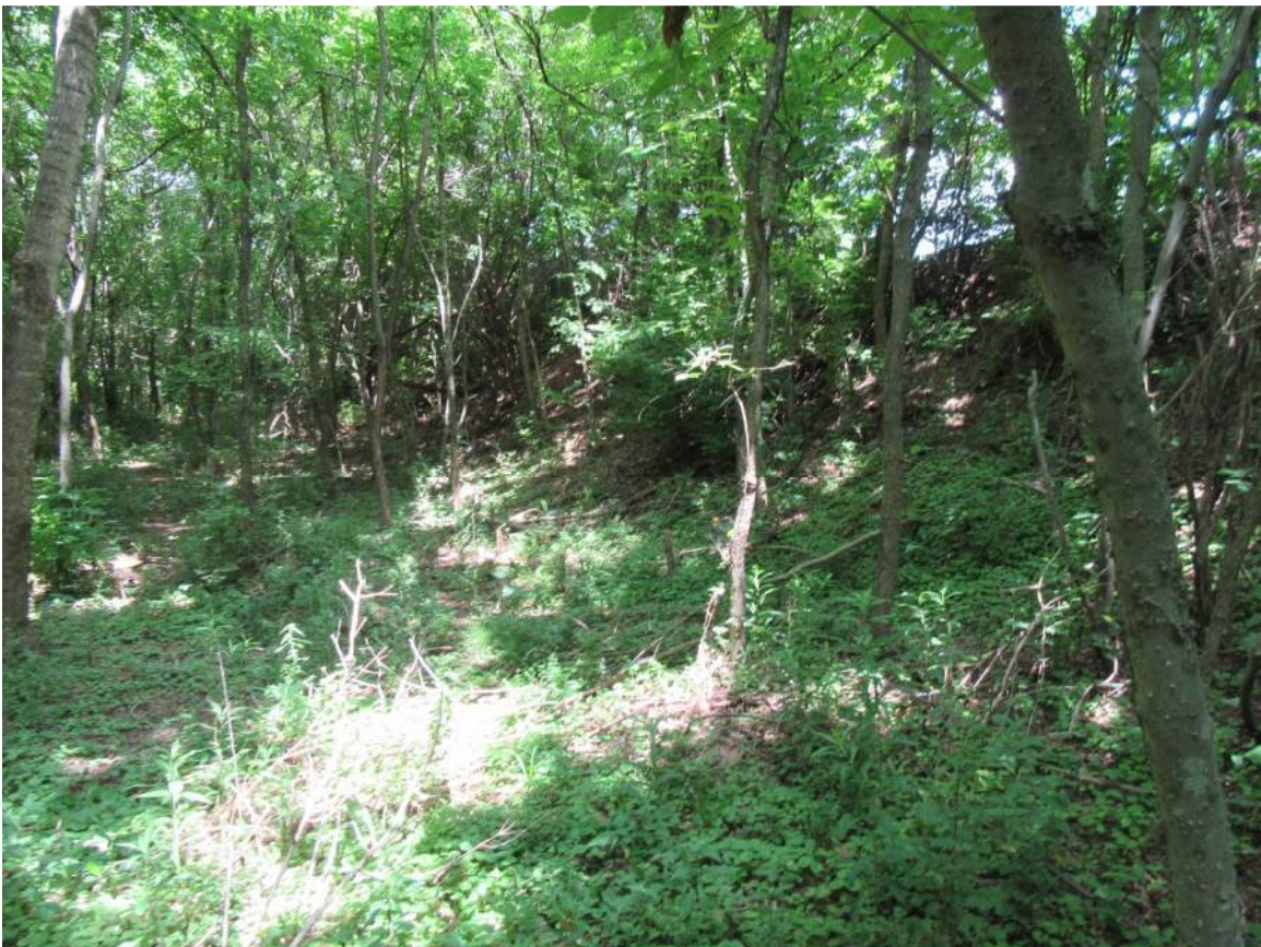
Photo No. 10: Downstream slope and downstream area viewed from left abutment.
