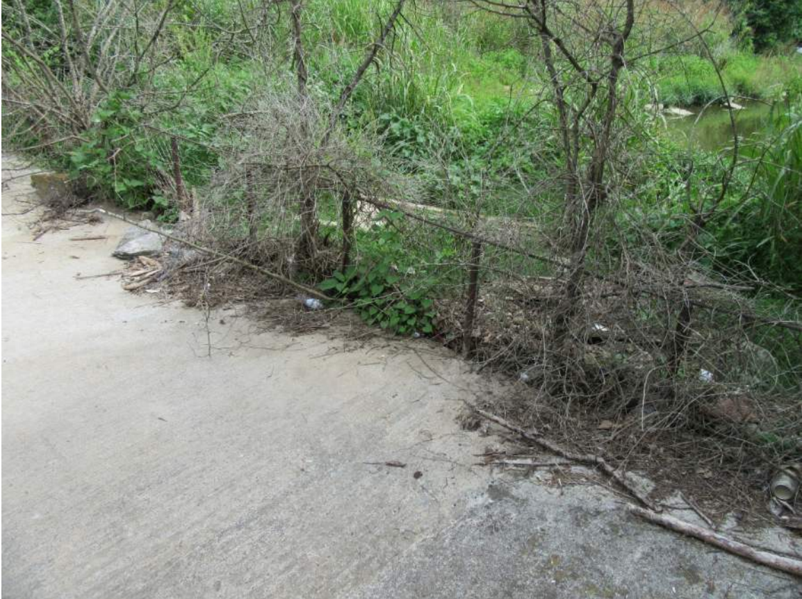
Photo No. 17: Fence (trash guard) on upstream side of spillway weir.
