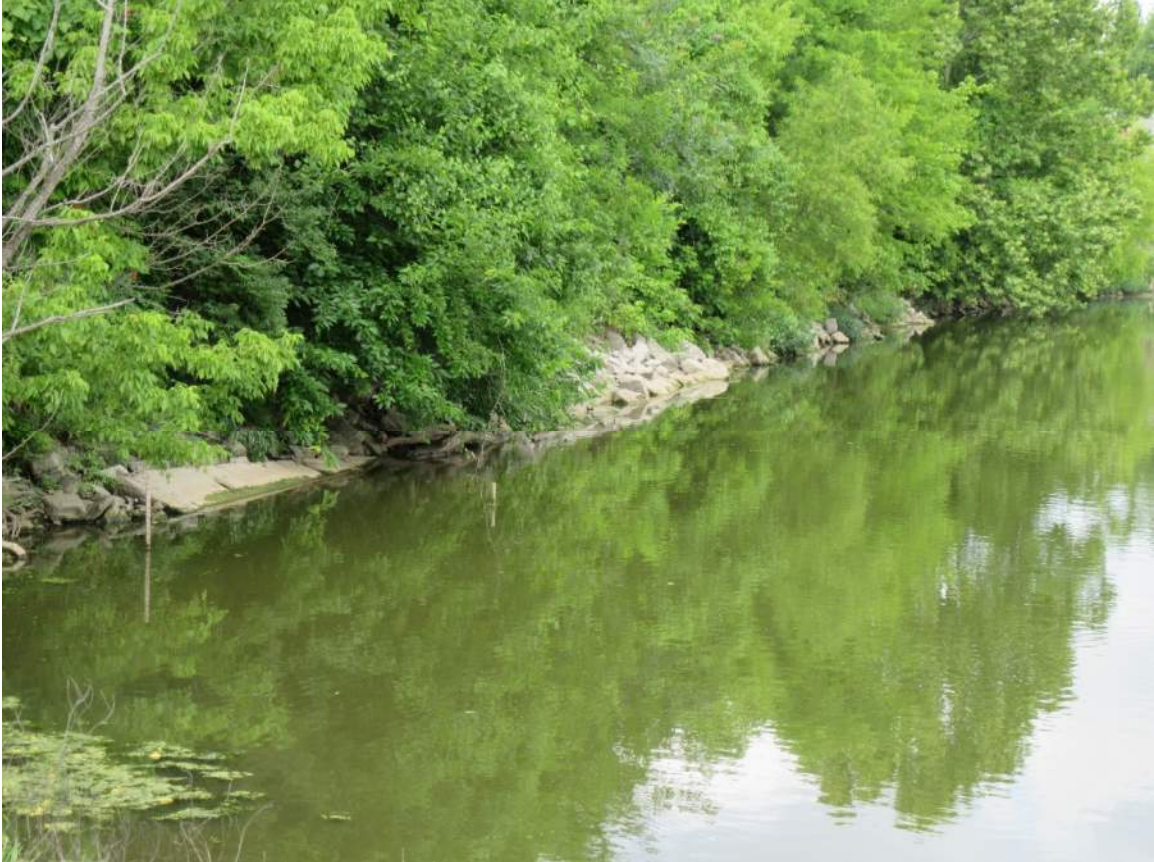
Photo No. 7: Riprap present on portions of upstream slope.
