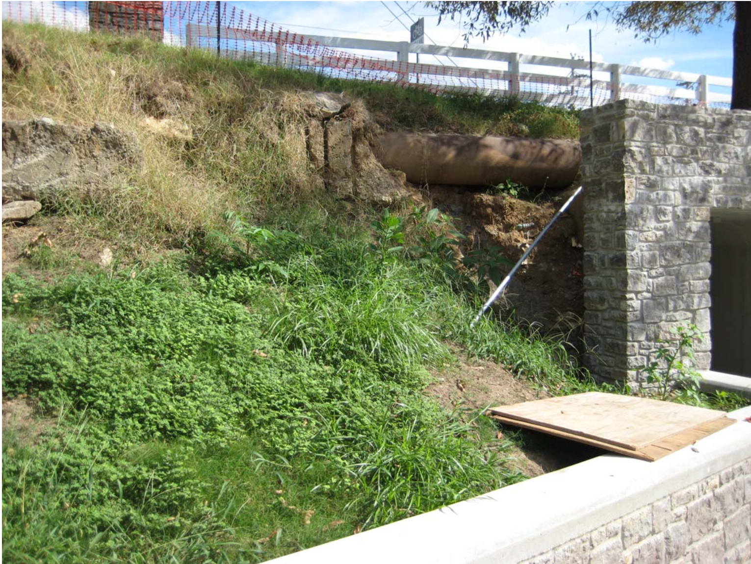
Looking Southeast at Steep Slope to North of Hillsboro Road Tunnel
