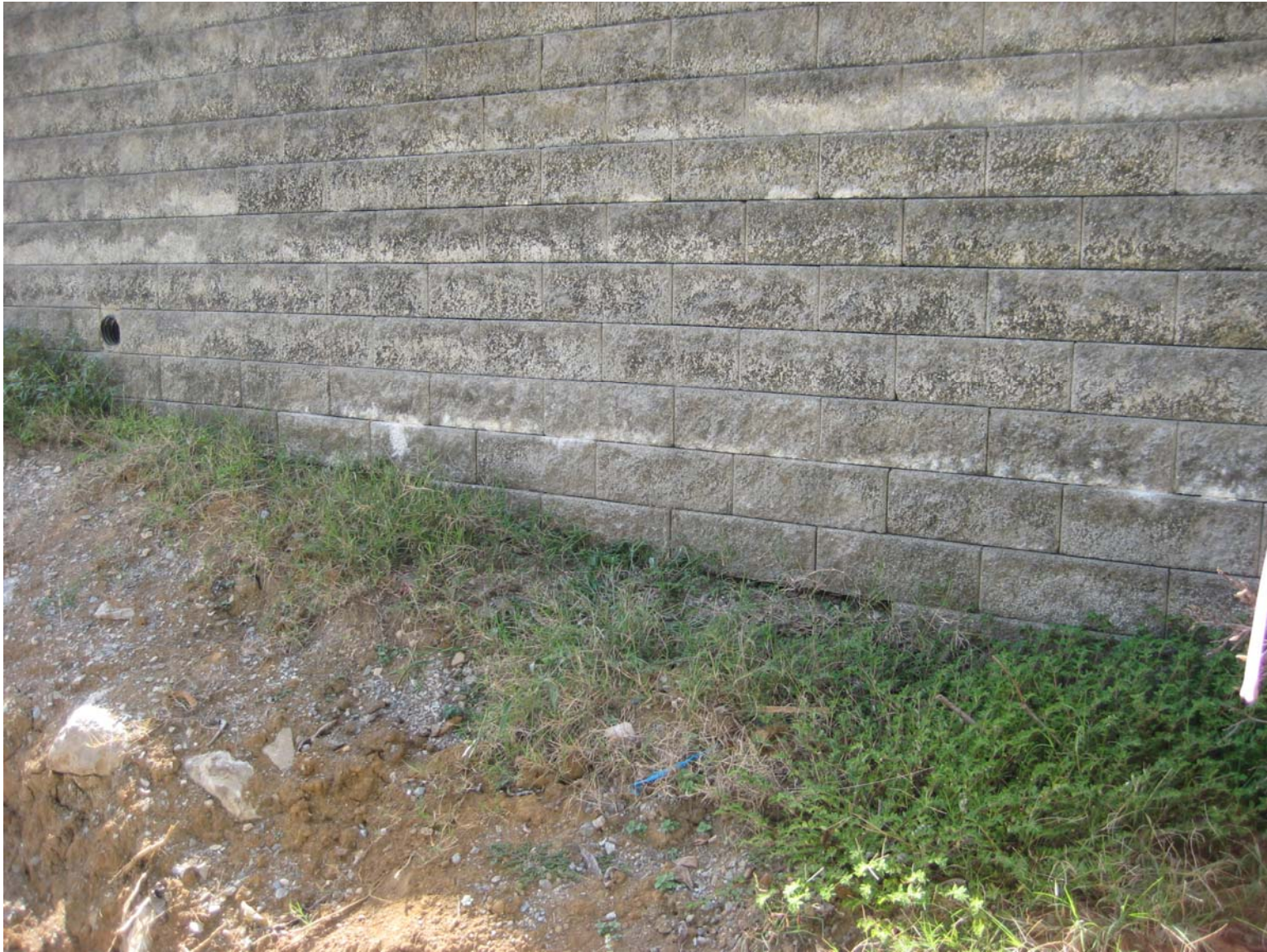
Close-Up View of Base of Existing Retaining Wall
