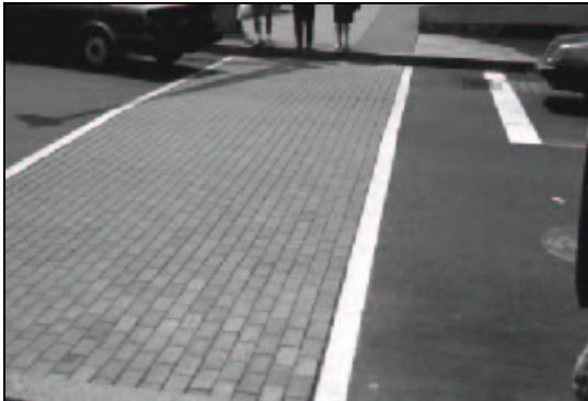
Figure 3-6 3-7: Example of a cross walk constructed of stenciled concrete. Pedestrian cross walks constructed of stenciled concrete, or an approved equivalent, enhance historic character CAO 2 and serve as a traffic-calming measure.
