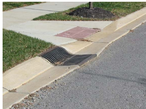
Rollover curb with grate transition
