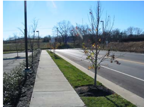
Typical Sidewalk with Grass Strip
