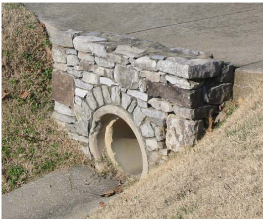
Protected Endwall with Stone Veneer
