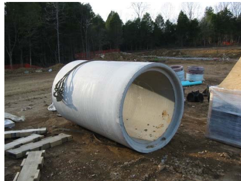
Reinforced concrete pipe is standard for city streets
