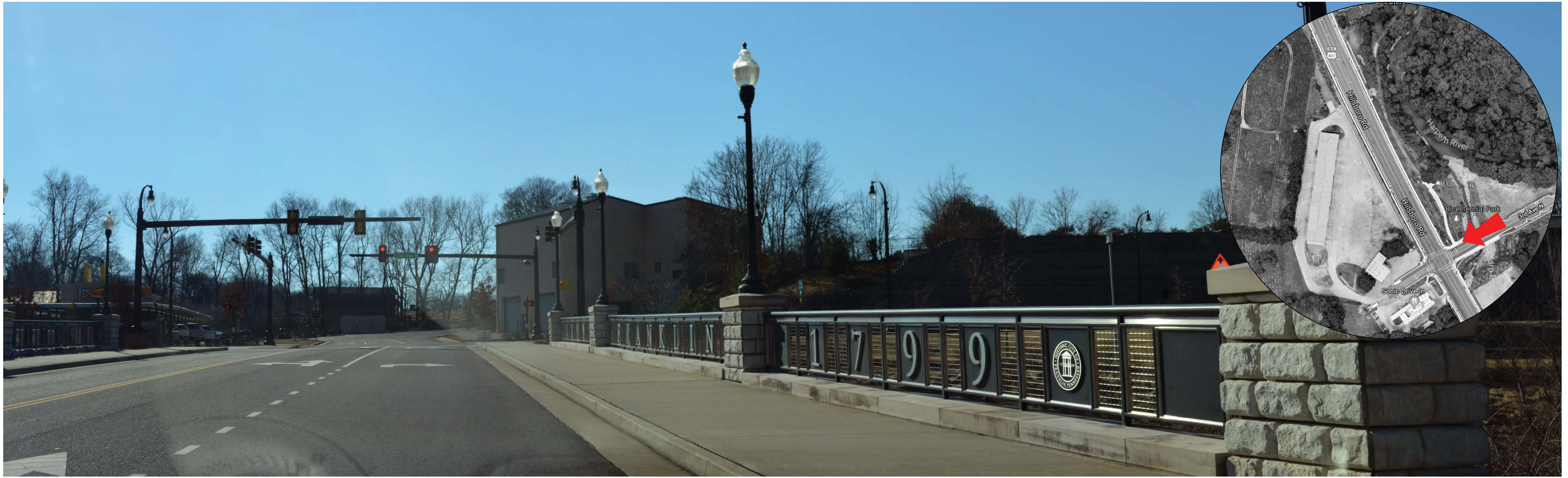
View from 3rd Avenue looking towards Hill Property
