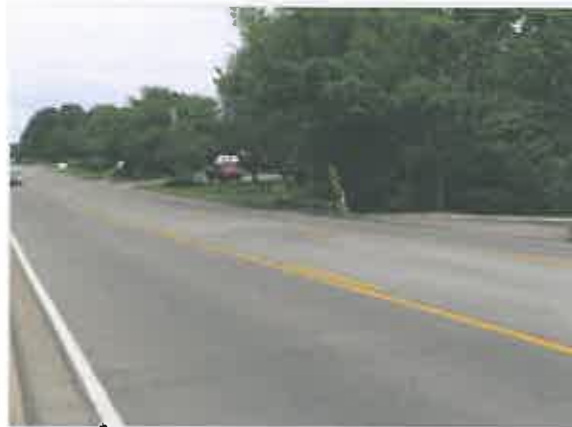
Seaboard Lane Streetscape Showing Lack of Sidewalks
