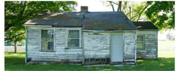
8 SOUTH WORKER HOUSE 2
