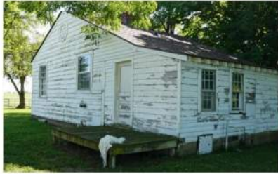
4 WEST WORKER HOUSE 1
