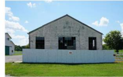
2 WEST POWER STATION
