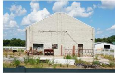
1 EAST POWER STATION
