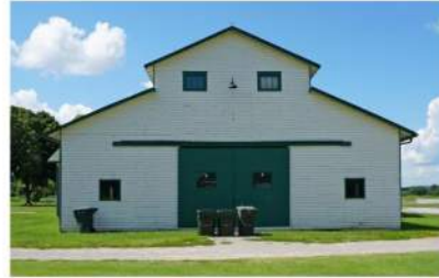
1 NORTH MAIN BARN
