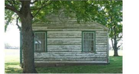
6 WEST WORKER HOUSE 2
