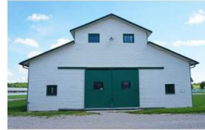
2 SOUTH MAIN BARN
