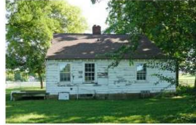
2 SOUTH WORKER HOUSE 1
