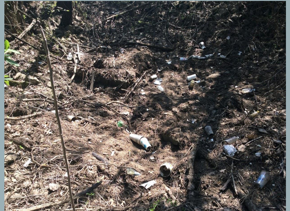
Jim Warren Park: Clean storm infrastructure
