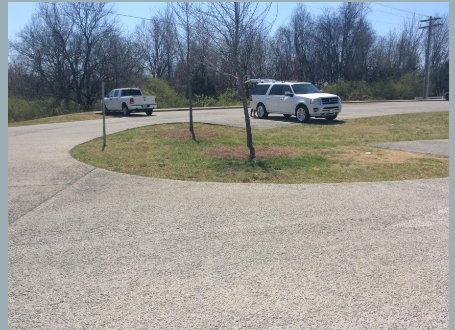
Eastern Flank pervious concrete
