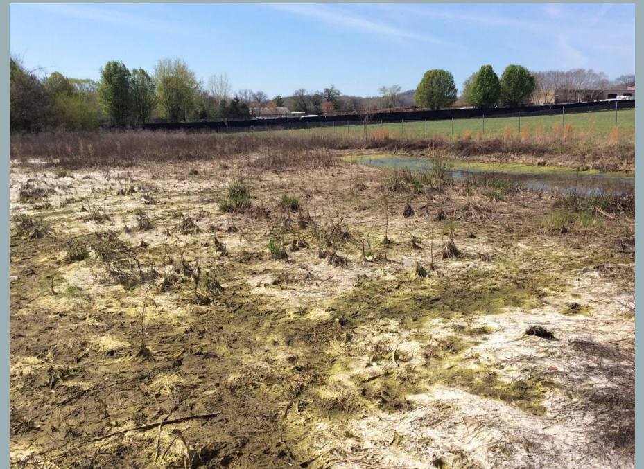
Public Works: Sand filter bed not installed
