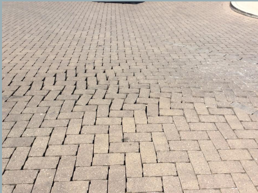
First Bank @ Five Points: Reinstall permeable pavers
