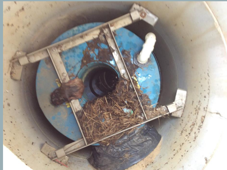
Fire Station #8: Clean water quality unit
