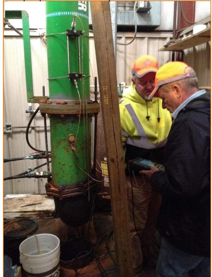
Figure 3. We utilize premium handheld acoustic units to listen to water services, hydrants, and ground microphone attachments to pin-point leaks for repair.
