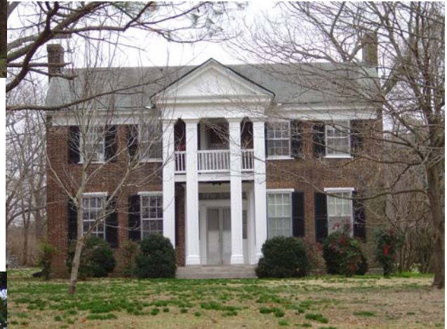
Thomas Shute House, "Creeside", National Register Property
