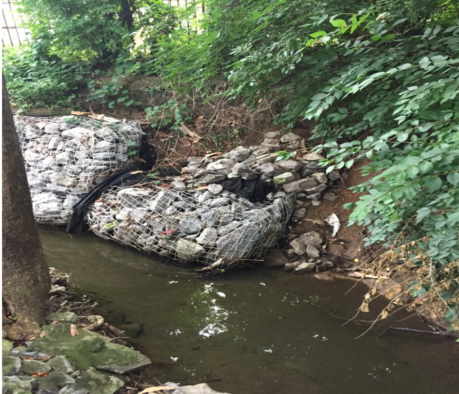
Photo 4: Failing toe of right descending bank in Reach 3.
