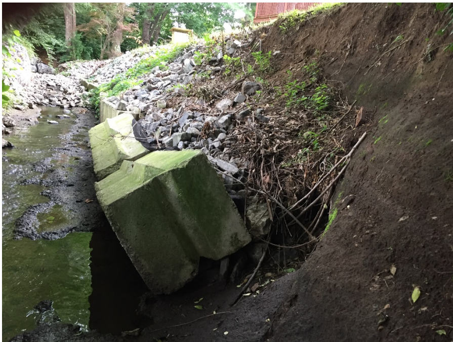
Photo 3: Failing toe of left descending bank in Reach 3.
