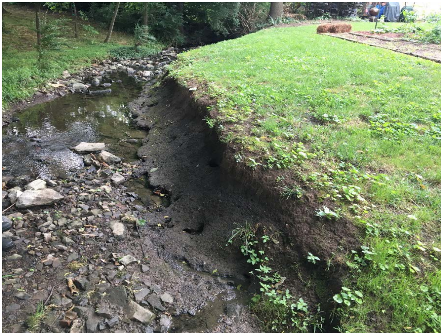
Photo 1: Reach 1 where right descending bank is eroding adjacent to a concrete swale draining water from the street.
