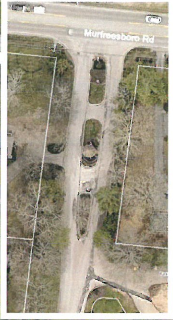
Subdivision Entrance, North Median, and Guard House
