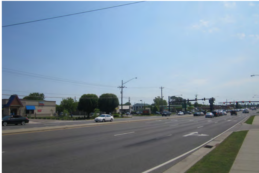
State Route 96 (Murfreesboro Road) is an example of a principal arterial street.
