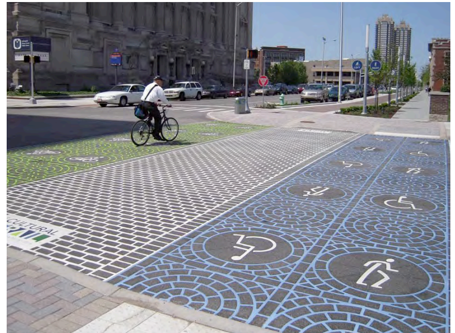
This highly visible stamped crosswalk also incorporates trail system identity.
