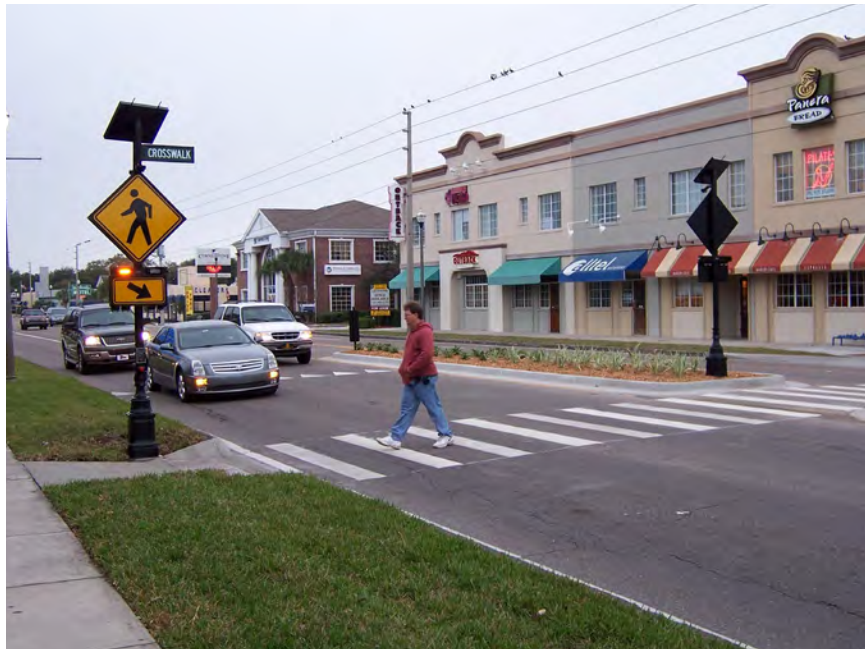
A Rectangular Rapid Flashing Beacon creates a more visible crosswalk.
