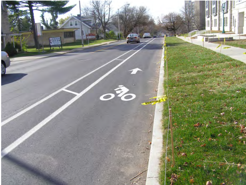
A buffered bicycle lane includes additional designated space separating the bicycle lane from the vehicle travel lane.
