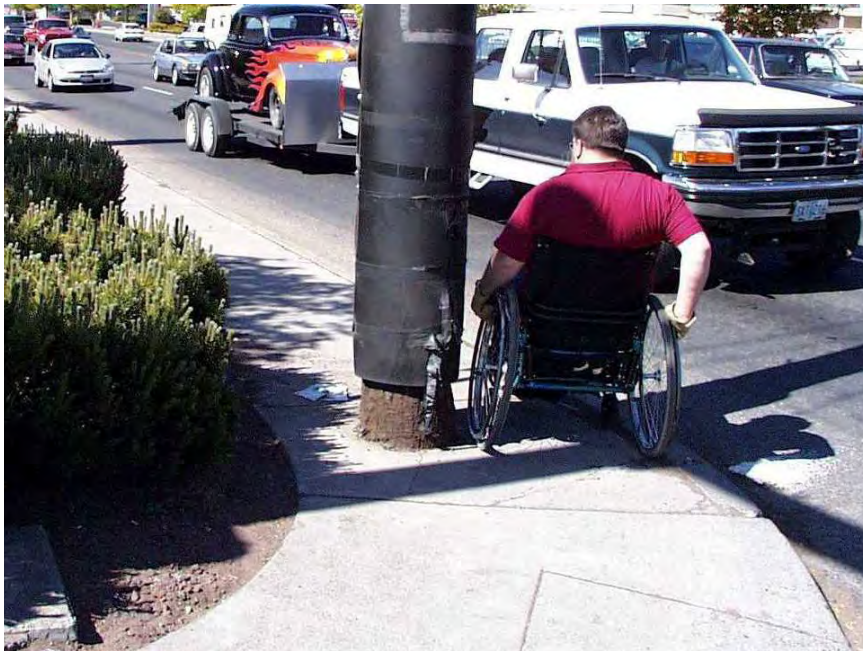
Utility poles in the sidewalk create significant barriers to accessibility.
