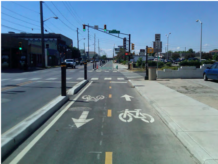
This two-lane cycle track is buffered from the adjacent road with a raised curb and bollards.
