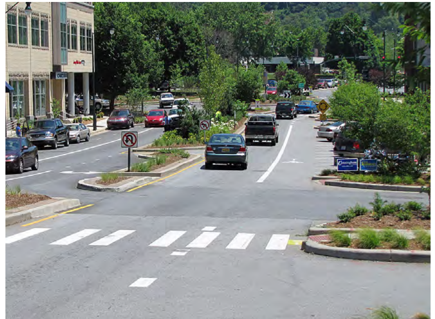
Curb extensions or “bump-outs” are used to shorten the crossing distance and can be used for aesthetics and stormwater capture.
