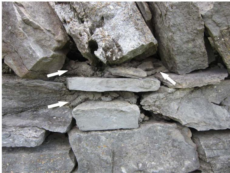
Figure 24. Evidence of hard Portland cement mortar in some areas of the walls.
