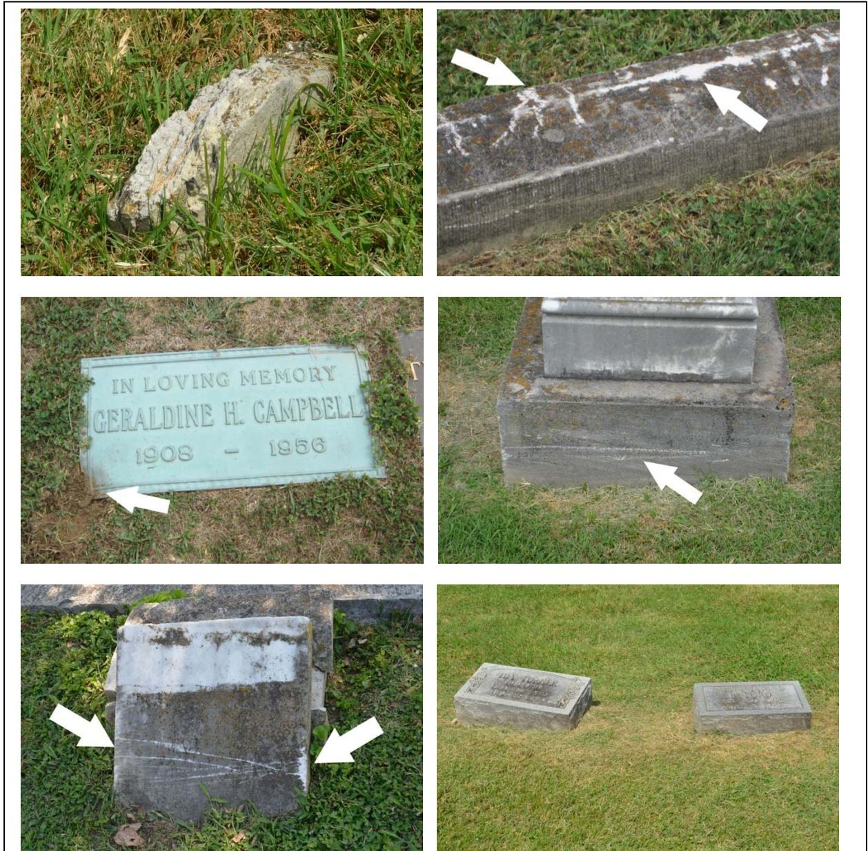
Figure 55. Mowing damage in Rest Haven Cemetery. Upper left shows a footstone repeatedly run over by mowers fragmenting and destroying the top. Upper right shows coping repeatedly impacted by mowers running over it. Middle left shows a bronze lawn marker damaged by a mower. Middle right shows a monument scraped by a mower. Bottom left shows both mower impacts and mower scrapes on a toppled monument. Bottom right shows a lawn marker displaced by mower impacts.
