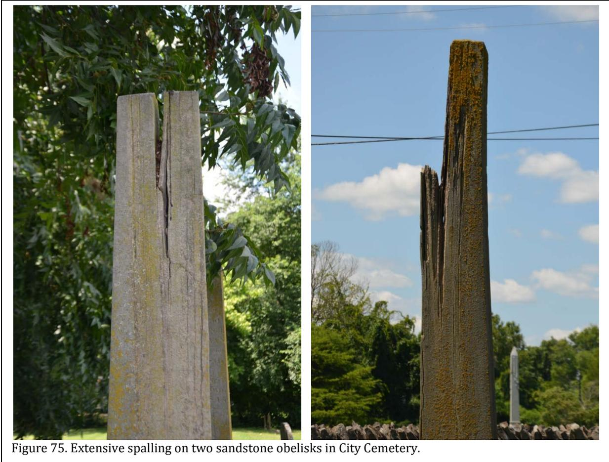
Figure 75. Extensive spalling on two sandstone obelisks in City Cemetery.
