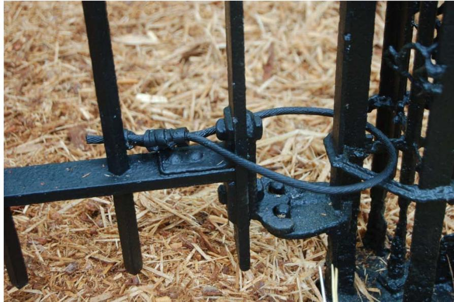
Figure 37. Example of a gate protected with stainless steel cabling that has been painted to blend with the fence.
