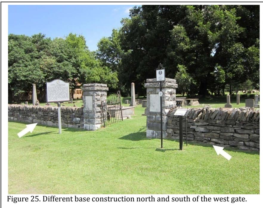
Figure 25. Different base construction north and south of the west gate.
